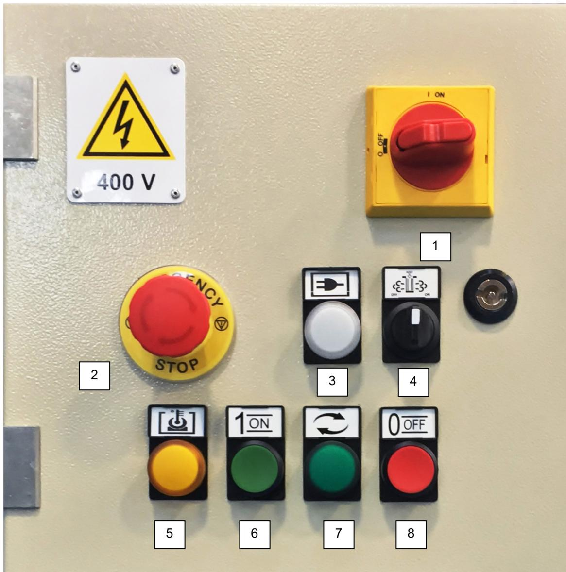
1. I / O switch: ELECTRIC PANEL POWER SUPPLY
