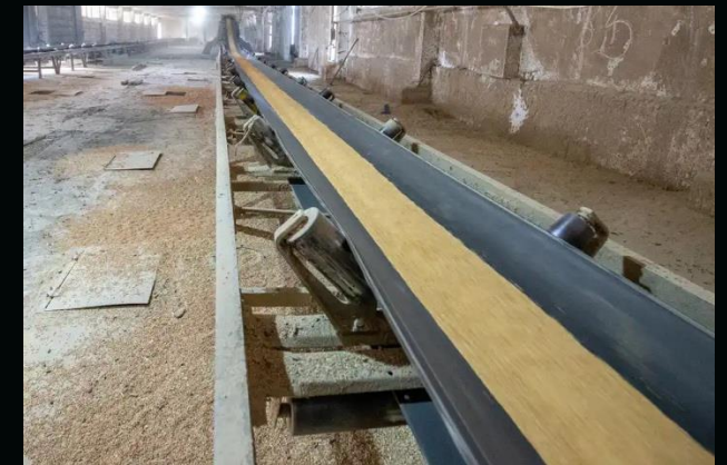
Conveyor belt tunnel detail
